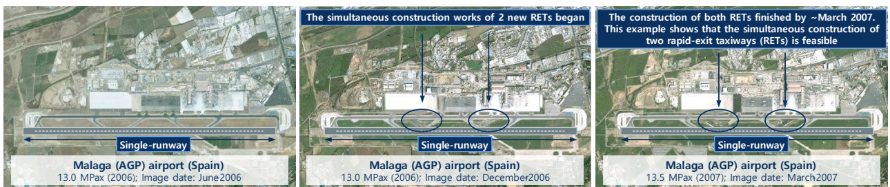
Figure 325: Simultaneous construction of two (2) additional rapid-exit taxiways (RETs) in Malaga (AGP) airport (example)
