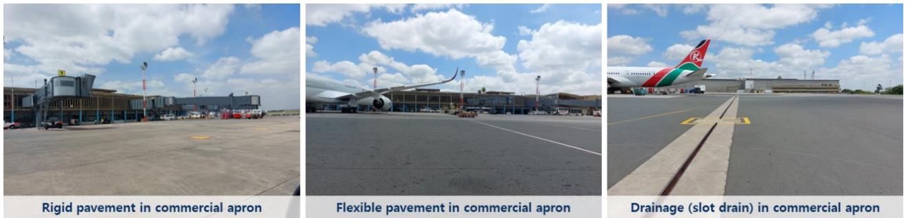
Figure 128: Apron snapshots from the site visit at JKIA
